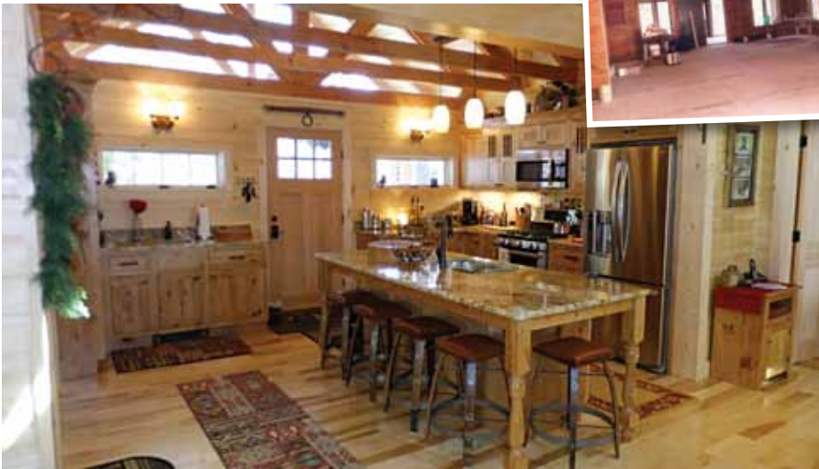
Both the owners and Lorraine felt that if anything besides the daylight basement was added it would no longer have that “camp” feeling. They did, however, raise the height of the kitchen by adding a gable peak of Douglas fir beams above it.
